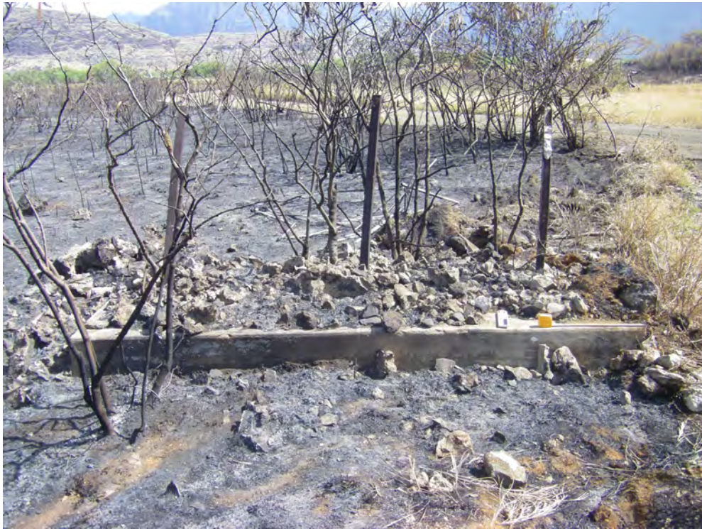
Photo 20. Feature 14, concrete pad. View north.
