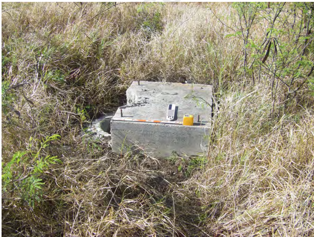
Photo 14. Feature 13, concrete pedestal foundation. View south.
