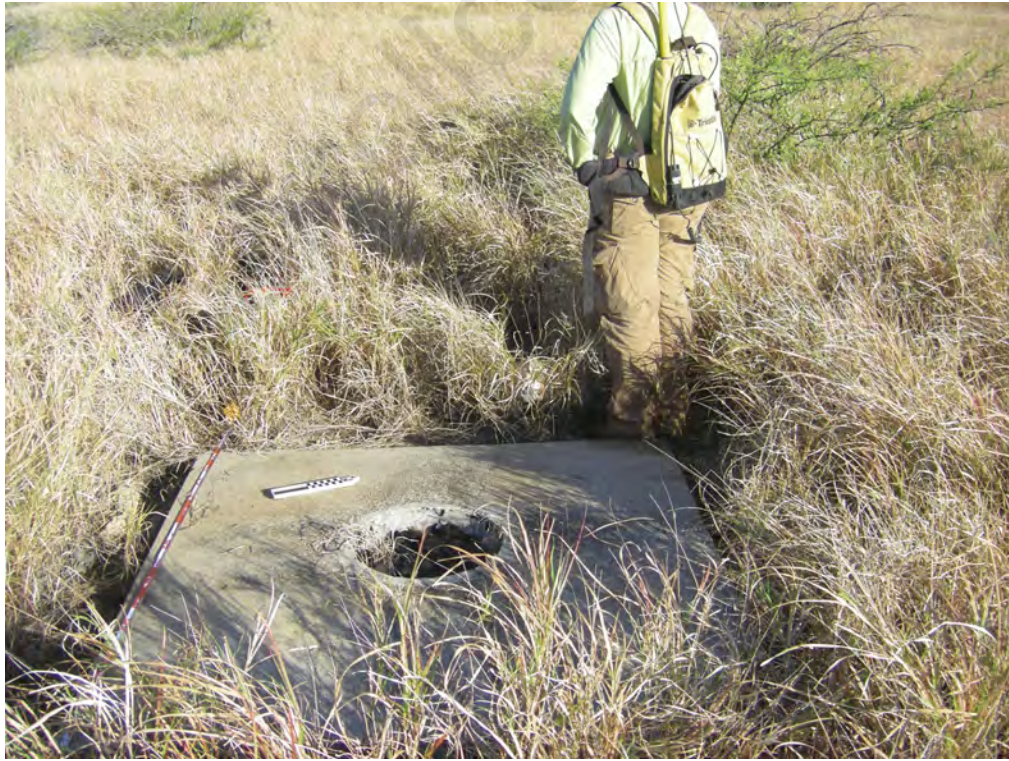
Photo 5. Feature 2, concrete pedestal foundation. View west.
