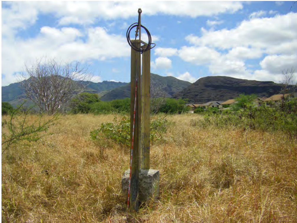
Photo 17. Feature 17, concrete pad foundation with metal support. View east.
