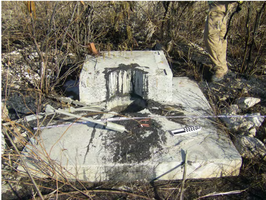
Photo 7. Feature 4, concrete pedestal foundation. View west.
