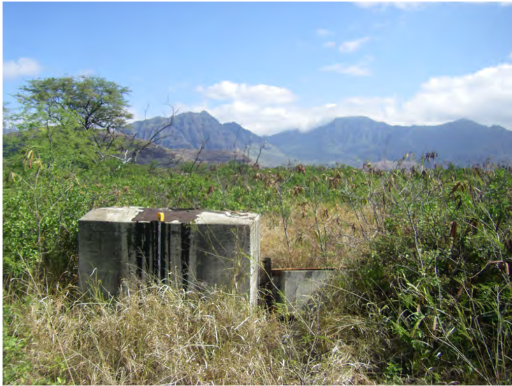
Photo 15. Feature 15, concrete pedestal foundation. View north.
