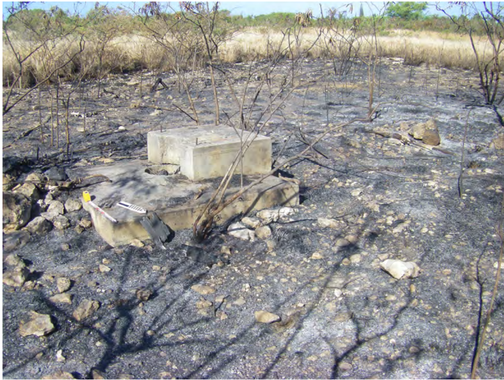
Photo 10. Feature 8, concrete pedestal foundation. View southwest.
