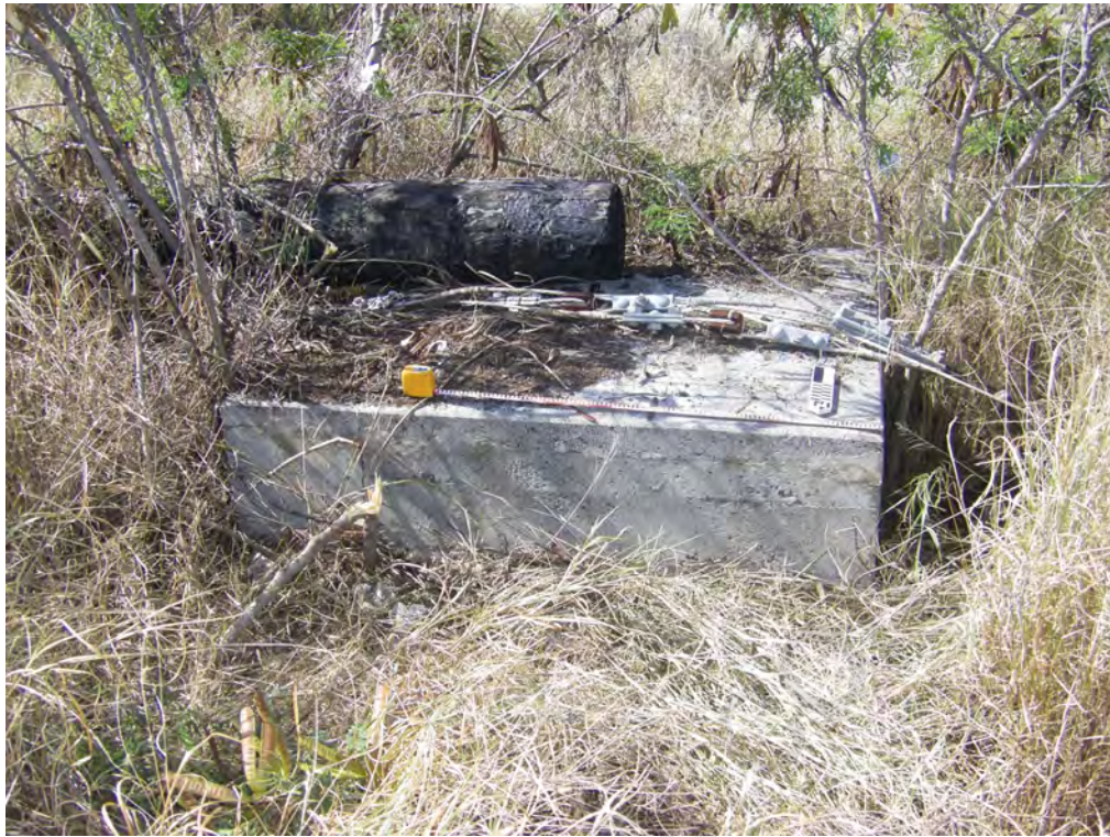
Photo 13. Feature 12, concrete pedestal foundation. View south.
