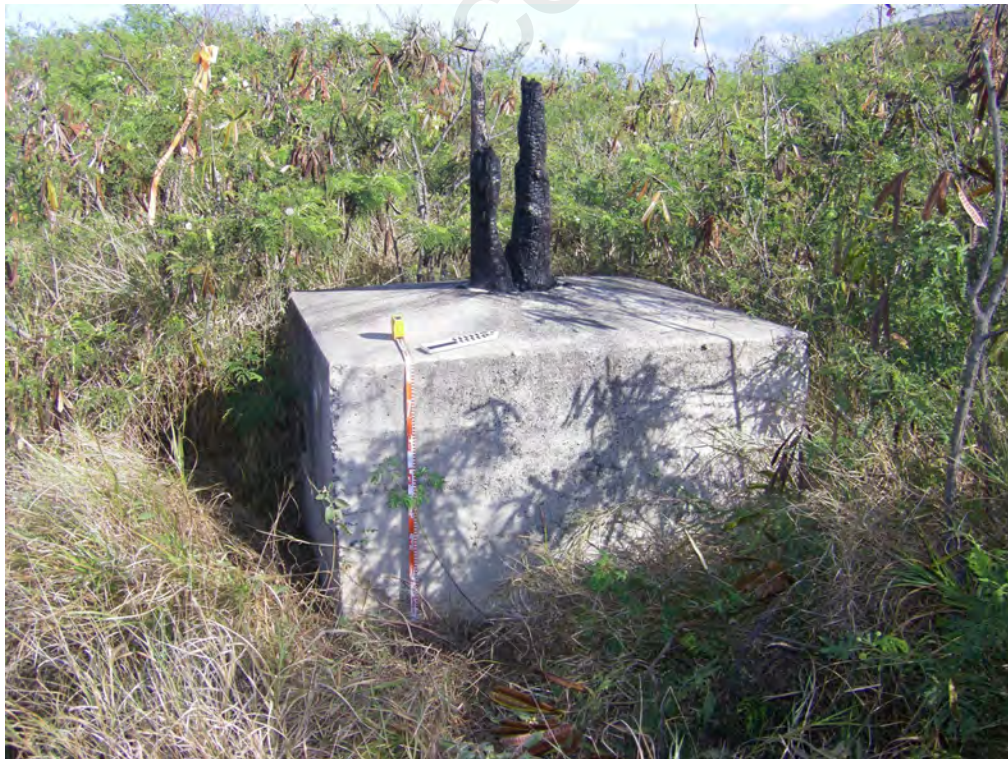
Photo 8. Feature 5, concrete pedestal foundation. View west.
