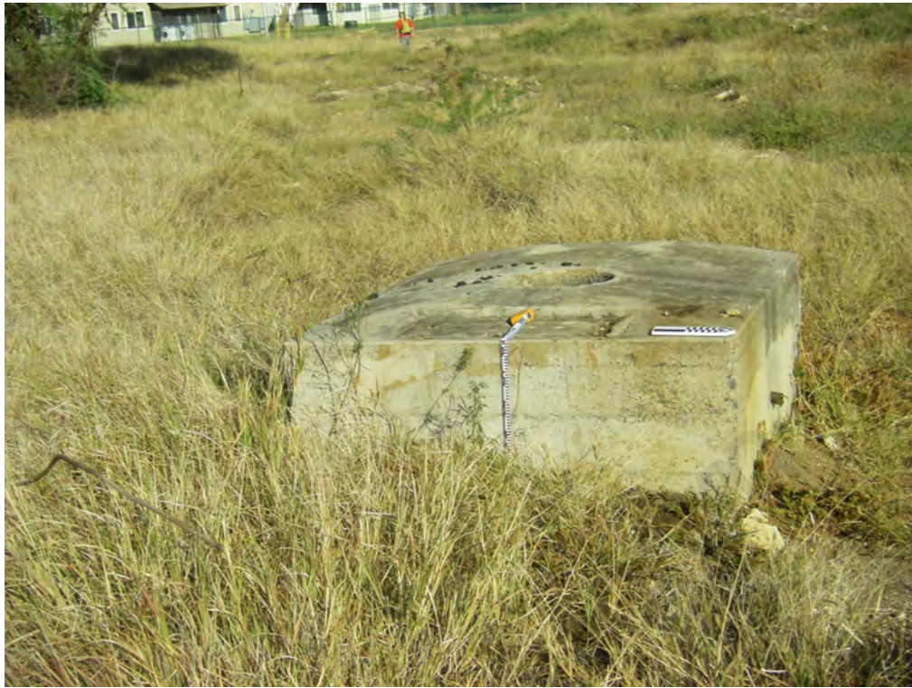
Photo 4. Feature 1, concrete pedestal foundation. View west.
