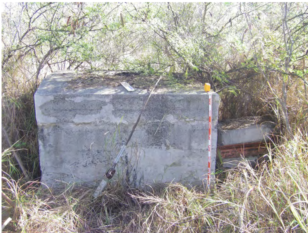
Photo 9. Feature 6, concrete pedestal foundation. View north-northeast.
