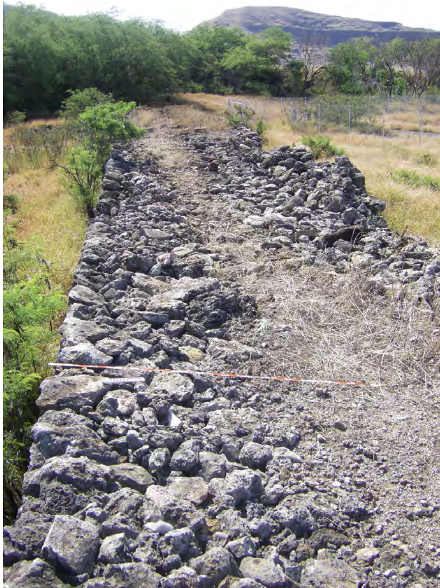
Photo 25. Feature 10, railroad bed, eastern segment. View east.
