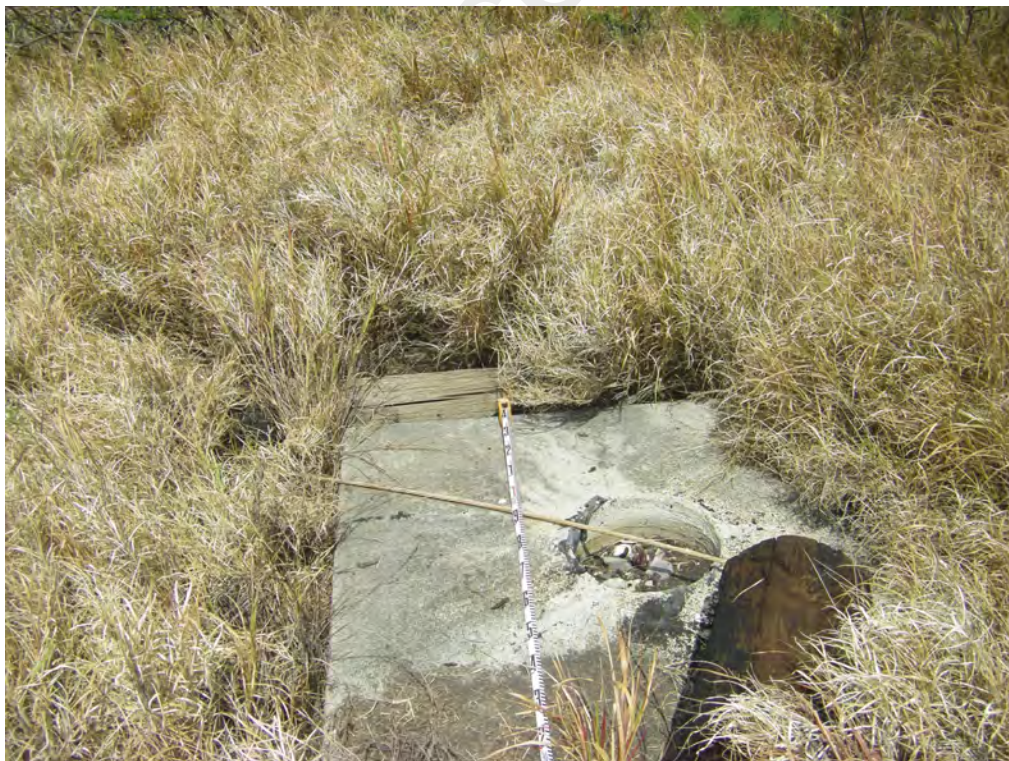
Photo 16. Feature 16, concrete pedestal foundation. View west.
