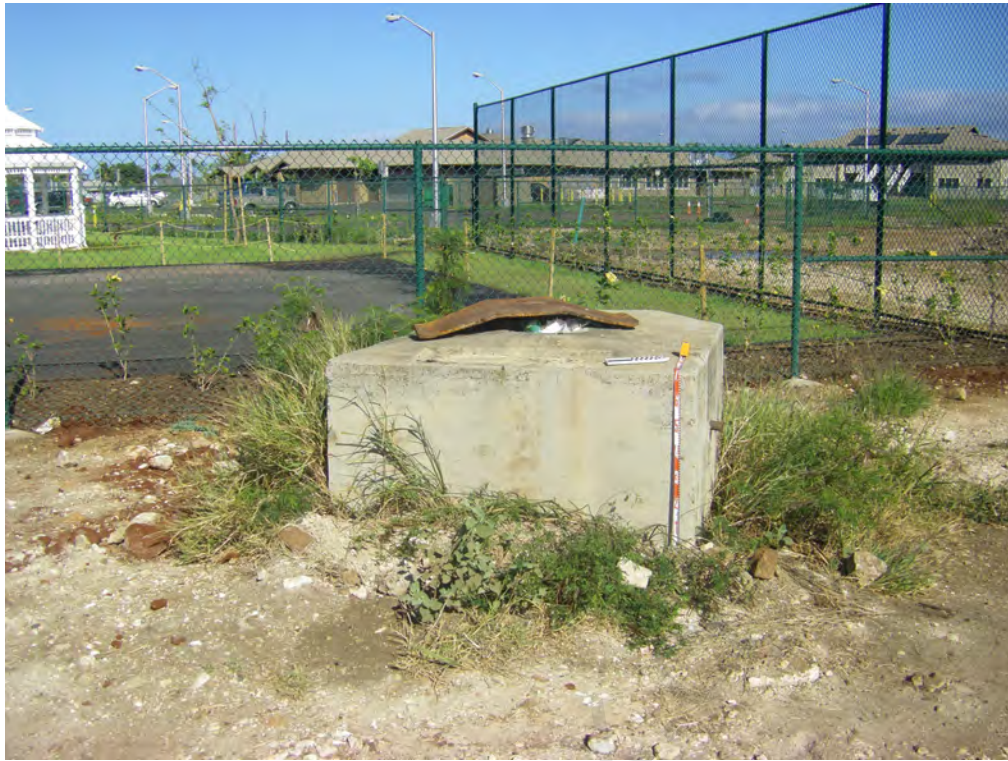
Photo 6. Feature 3, concrete pedestal foundation. View west-northwest.
