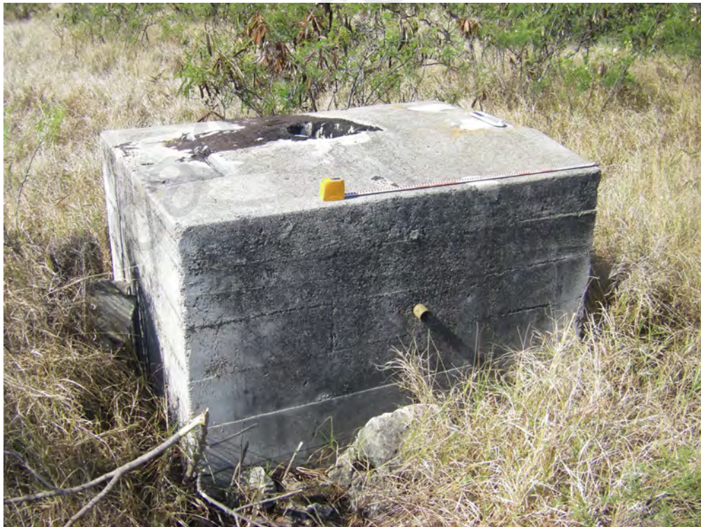
Photo 11. Feature 9, concrete pedestal foundation. View southwest.
