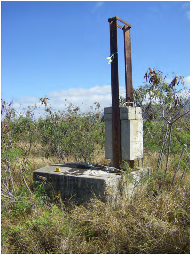
Photo 12. Feature 11, concrete pedestal foundation. View northwest.
